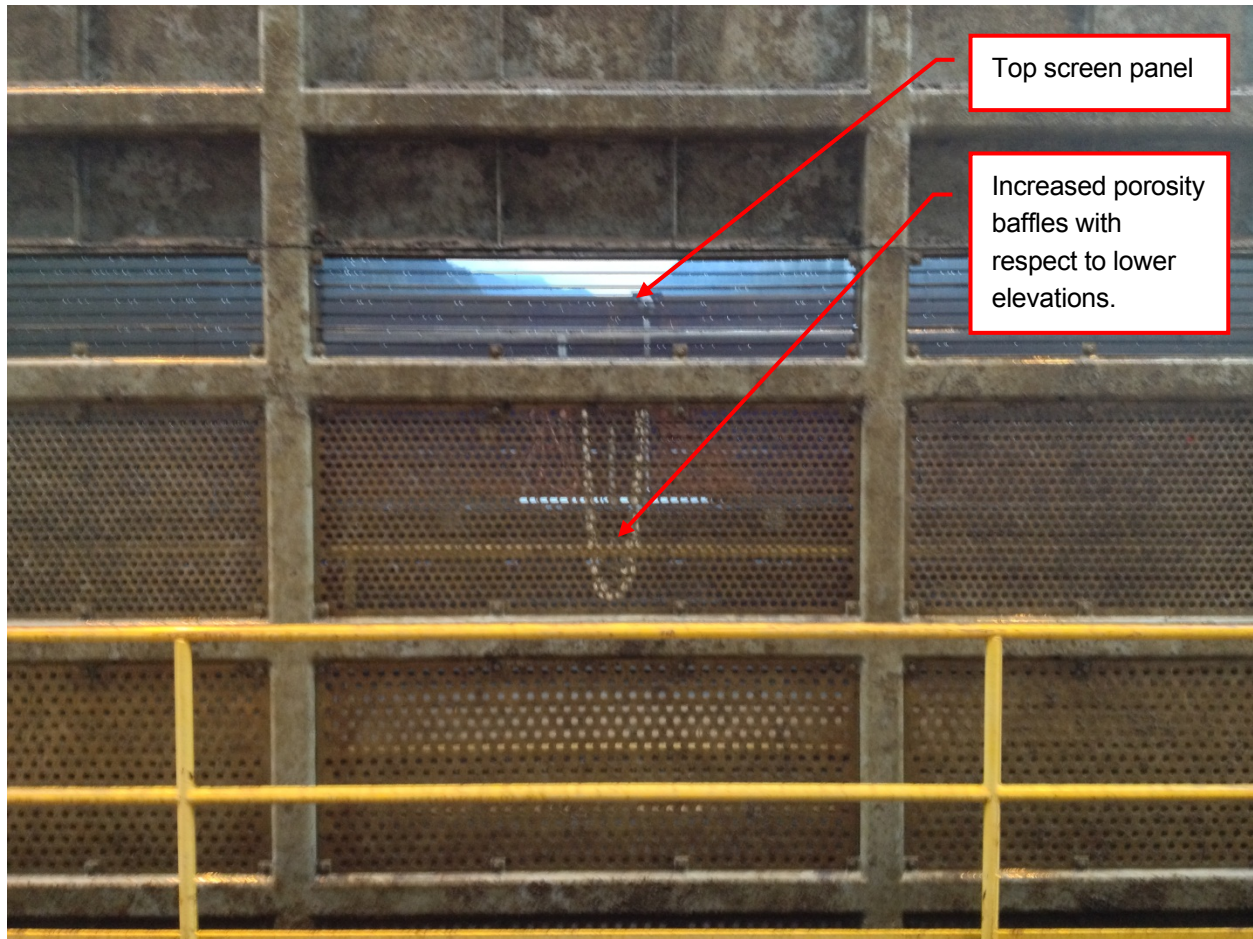
Photo 4-4 Top Unbaffled Screen Panel on VBS
