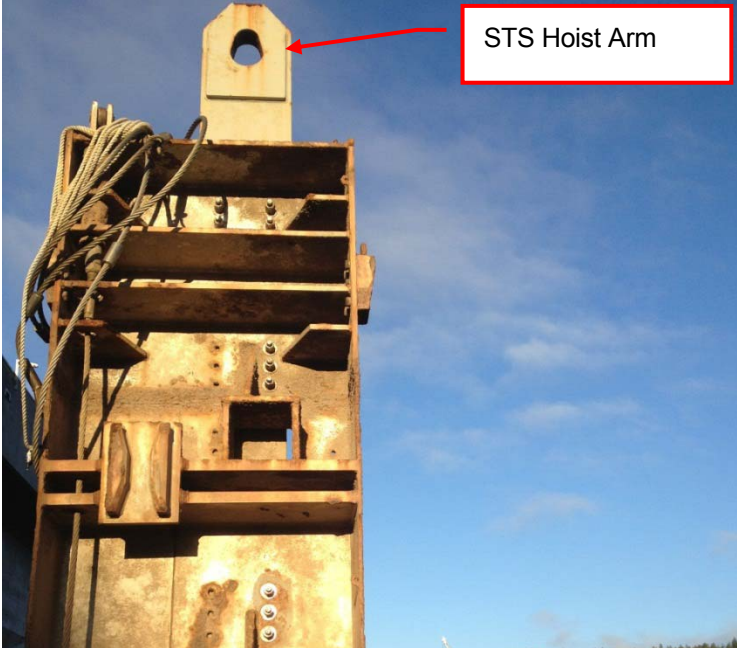
Photo 4-1 STS Hoist Arms
